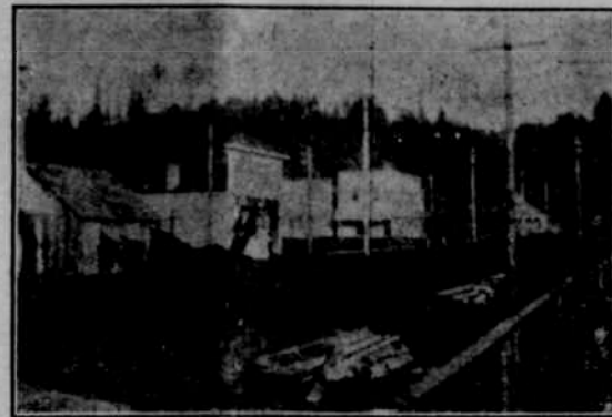
Second Street looking from Broadway to Main. The lumber seen is for sidewalk and the street
