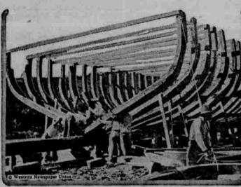
The shipyards of Cuba have been scenes of much activity since Cube entered the war. The construction of wooden ships, so as to release steel ships for war requirements, is going on without delay. The photograph shows one of the wooden ships under construction.
