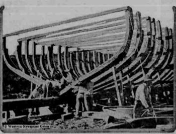
The shipyards of Cuba have been scenes of much activity since Cubi entered the war. The construction of wooden ships, so as to release ships for war requirements, is going on without delay. The photograph shows one of the wooden ships under construction.
