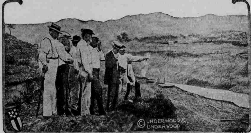
The great slides which have blocked the Panama canal have become a matter of such concern to the United States that President Wilson appointed a commission to study the causes of the slides. The photograph shows General Goethals and the commission viewing the slides and watching boats go through the canal.
