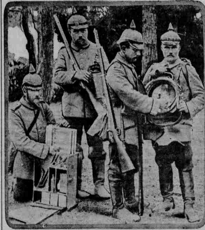
Among the many devices with which the German army is equipped is this portable searchlight, small but powerful, which, when not in use, is taken apart and distributed among five men.
