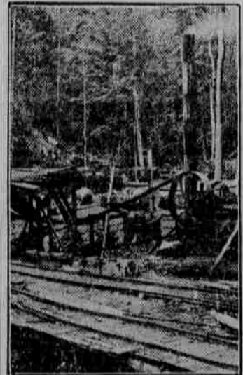
A Typical Small Portable Sawmill, Cutting About 4,000 Board Feet of Lumber a Day—Located Near Cumberland, Tenn.
