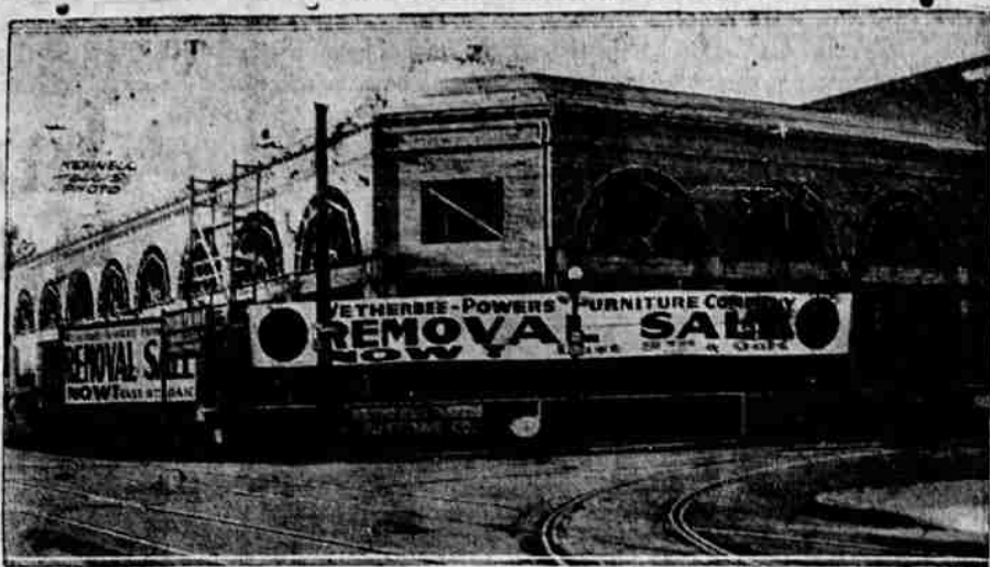
Wetherbee-Powers Building Nearly Completed
