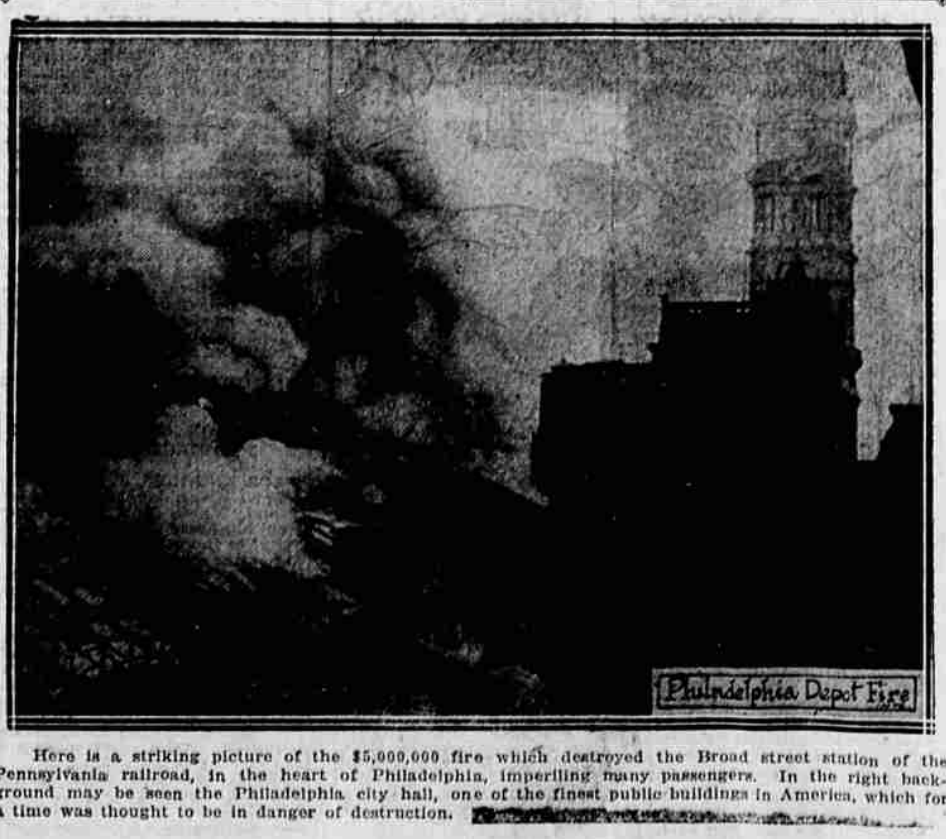
Here is a striking picture of the $5,000,000 fire which destroyed the Broad street station of the Pennsylvania railroad, in the heart of Philadelphia, imperiling many passengers. In the right background may be seen the Philadelphia city hall, one of the finest public buildings in America, which for a time was thought to be in danger of destruction.
