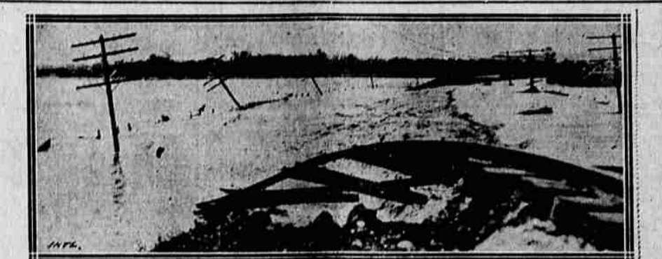
More than 20 lives were lost, and property valued at millions of dollars swept away when the Trinity river flooded a vast area between Fort Worth and Dallas, Texas. Heavy rains caused the rise in the stream. This first picture from the flood territory shows the tracks of the Houston & Texas Central railroad being washed away near Ferris, Texas.
