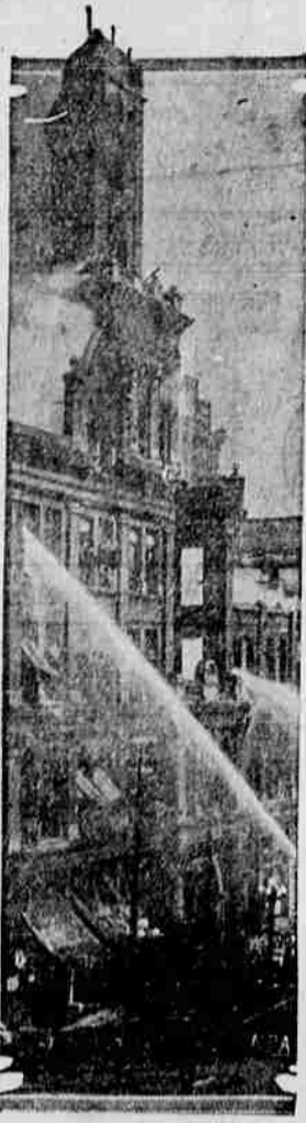
Several firemen were injured and property damage of $1,000,000 was sustained when the city hall at Birmingham, Ala., was destroyed by fire. The public library, housed on the top floor, was a complete loss.
