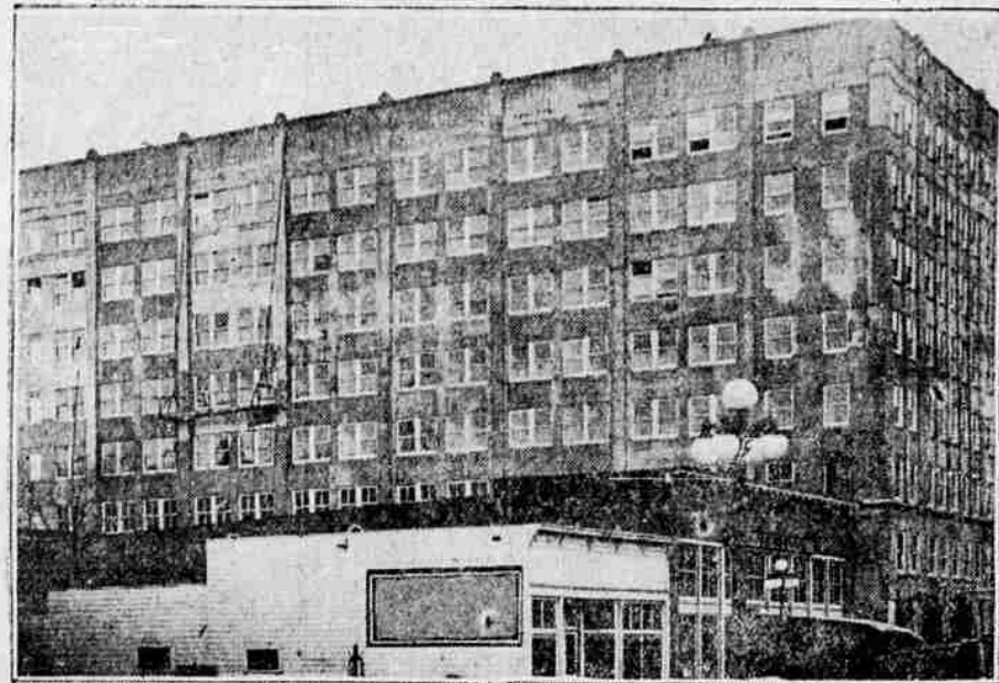
The W. E. Miner building, into which several tenants have already moved, is now receiving the finishing touches in its construction. It has taken just a year to build. A force of 100 men, under the direction of the W. W. Head construction company has worked on it steadily. It is 160 by 60 feet in size, and its eight stories contain 300 rooms. It is Eugene's tallest structure.
