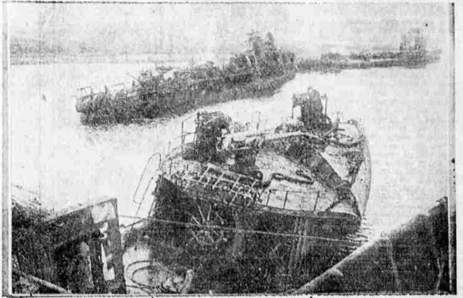
Salvaging Fleet Scuttled By Germans At Scapa Flow To Get Machinery, Brass And Copper Tubing
