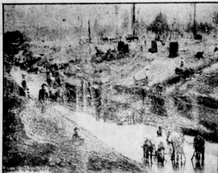
DIGGING THE DITCH.
