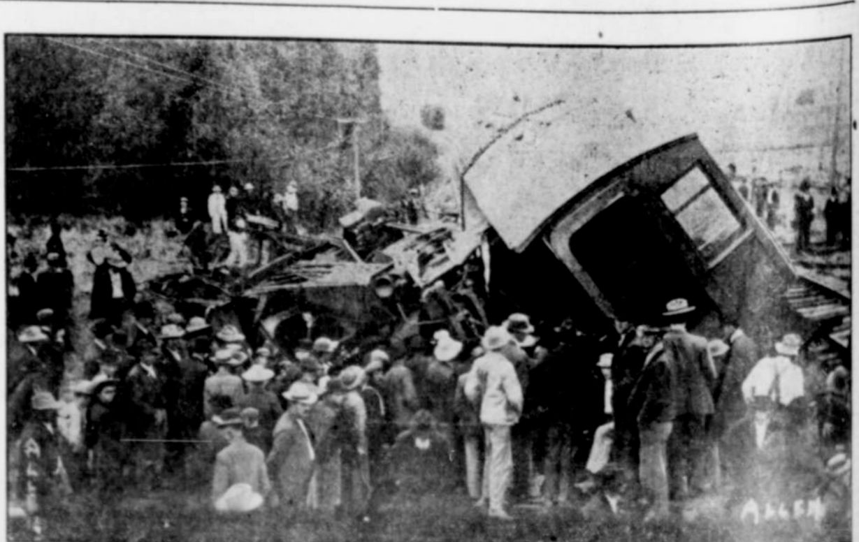
VIEW OF S. P. TRAIN WRECK AT IRVING
