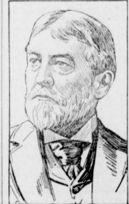
SENATOR EUGENE HALE. Chairman of the senate committee on naval affairs, which investigated criticism on the construction of our war ships.
