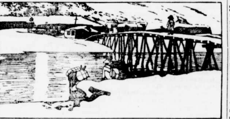
The bridge herewith illustrated leads from the Japanese settlement in Gensan, Korea, to the main town. Gensan is one of the most important seaports on the eastern coast of Korea.
