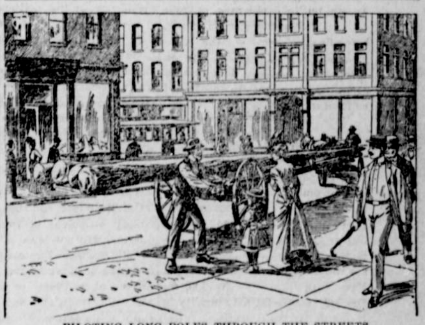
PILOTING LONG POLES THROUGH THE STREETS.
