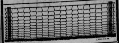
The Keystone Fence is made of good, strong wire and it is a continuous and entirely interwoven fence. This means that there is no beginning and no end to the stays, but that they are continuous with the long wires. And the stay wires will not slip and are not made of scraps.
