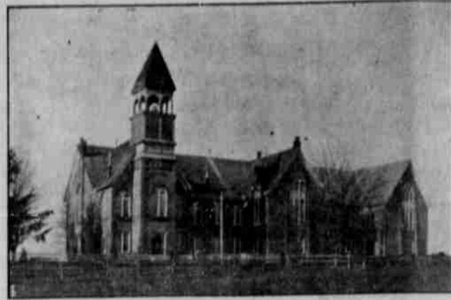
State Normal School Building.
