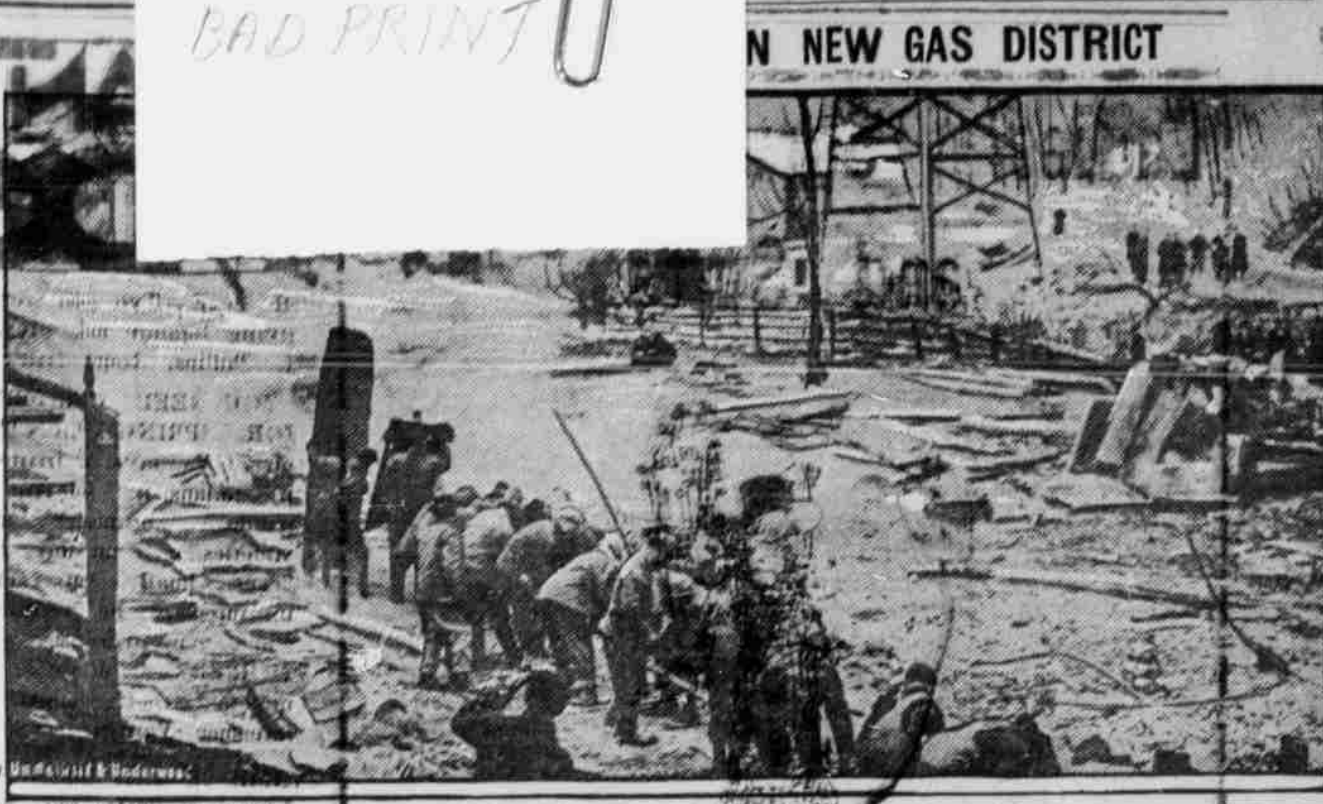
Men fighting a gas well fire at Snake Hollow, just outside Mead, Pa., where vast quantities of natural gas have been discovered recently. The men with the long pipe are trying to knock the cap off the well so the fire can be extinguished with steam.
