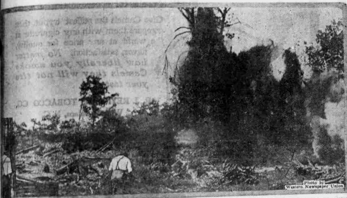
At Newark, N. J., a small army of men is busily engaged in clearing Heller field which, when completed, will be the first United States aerial mail landing field in the country. Our photograph shows the moment of detonation of a charge of dynamite beneath a mighty tree stump, which is torn from the grounds, roots and all.
