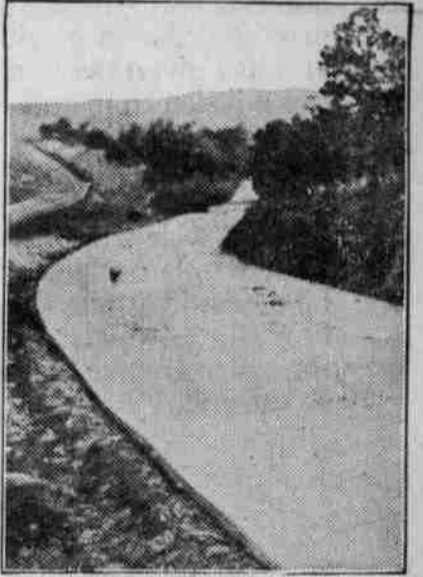
Concrete Road in Suburbs of Chicago.
