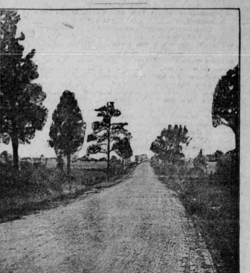
The Illustration Shows a Modern Oyster Shell-Macadam Road Between East Newmarket and Mt. Holly in the State of Maryland.
