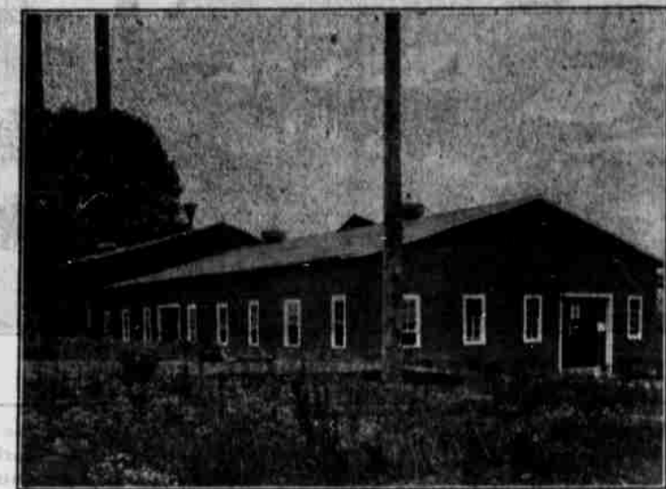
Electric Light Plant of Oregon Power Co.
