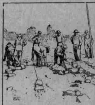
LAYING A TELFORD FOUNDATION
