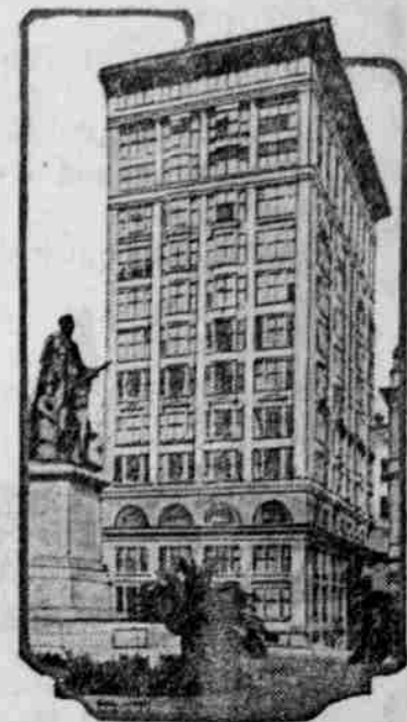
Above is shown the first ferro-concrete apartment house in Australia, located in Macquarie street, Sydney, which was recently opened by Premier George Fuller. There are 52 co-operative apartments in the building.
