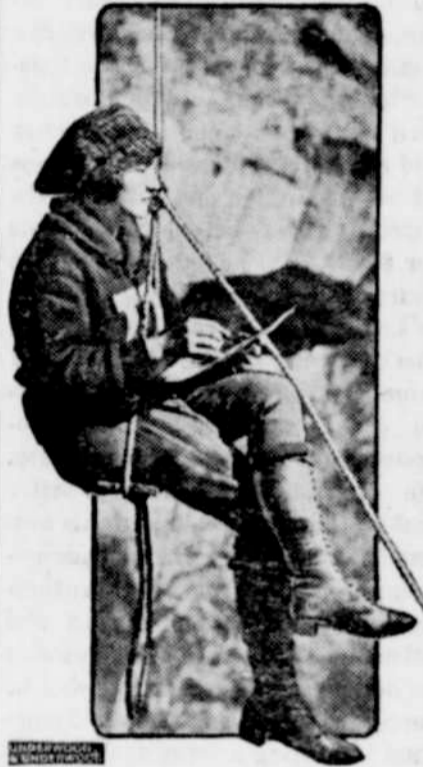
Eager to sketch cliff dwellings and to catch the exquisite colorings of canyon walls, Miss Dora Montague of Salt Lake City allows herself to be swung from dizzy heights on a narrow board seat. The photograph shows her sketching while swinging over a sheer drop of hundreds of feet in Zion National Park, Utah.
