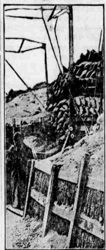
Entrance to a Dugout.
