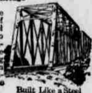
Built Like a Steel Bridge
