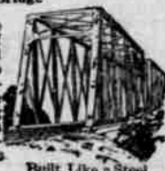
Built Like a Steel Bridge
