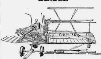
Supported Reel Chain Drive, Improved Canvas Tightener, Plenty of Binder Clearance, Has Three Packers instead of Two, Well Balanced and Light Draft.
