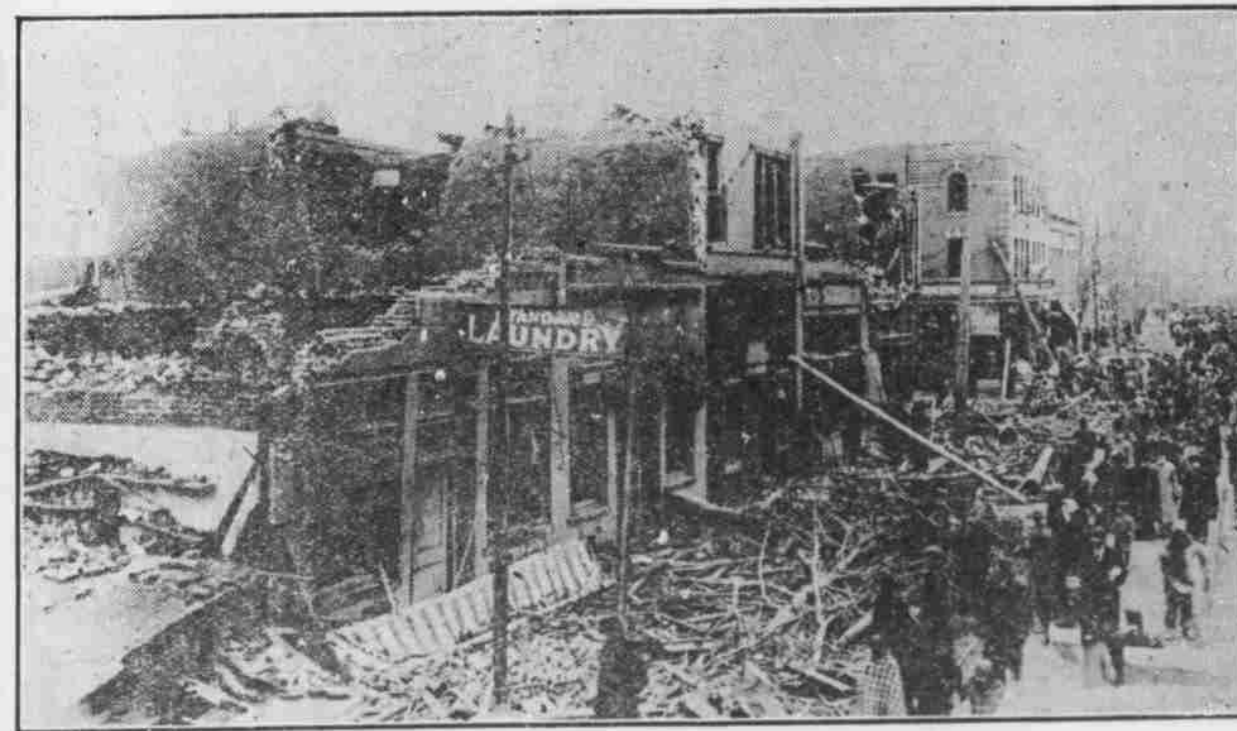
Photo copyright, 1913, by American Press Association. This picture was made within a few hours after Omaha had been wrecked by the tornado. It shows the appearance of Lake street at the intersection of Twenty-fourth. Not a building was left here with its roof intact, and many walls were blown down.
