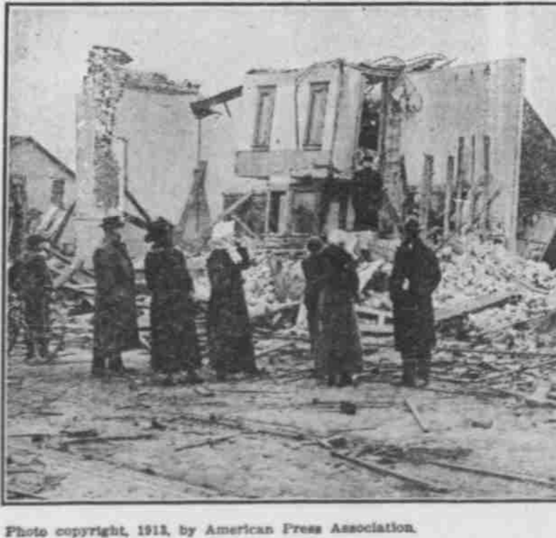
Photo copyright, 1913, by American Press Association. This photograph shows what was left of the Diamond moving picture theater after the storm had passed through Omaha. The loss of lives here was heavy. Many bodies were not recovered for days because of the delay due to a snowstorm.
