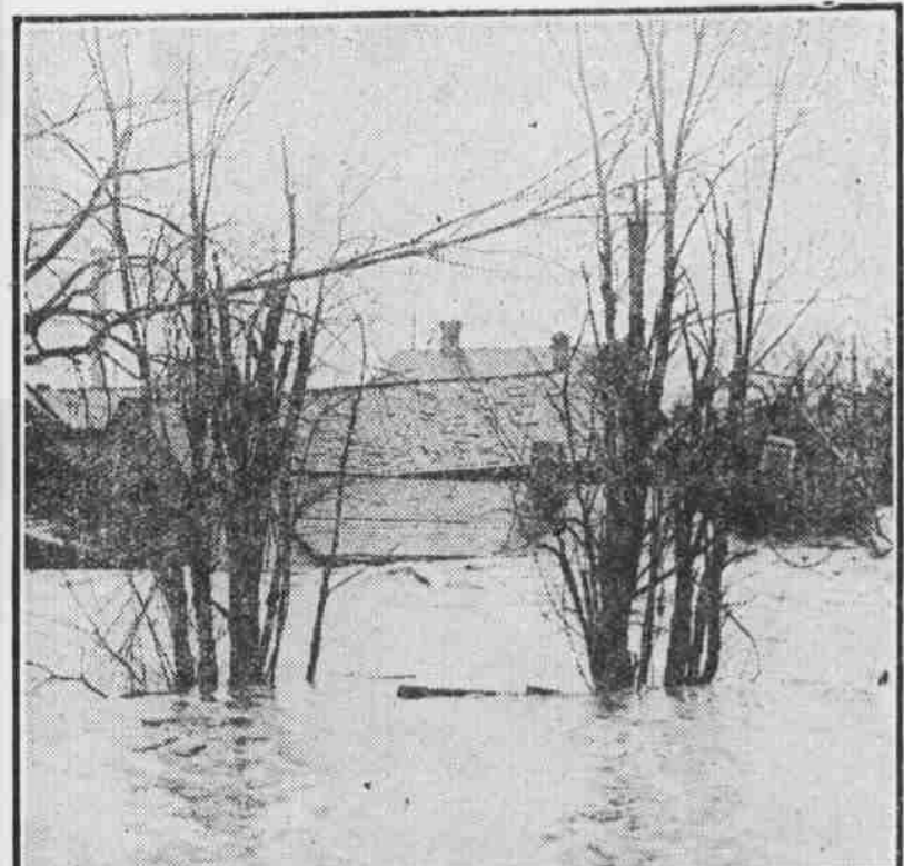
Photo copyright, 1913, by American Press Association. Many houses in Dayton were swept from their foundations to be hurled against other buildings by the water which swept through the streets as if through a millrace.
