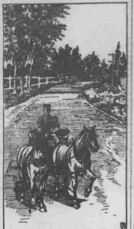
ROAD SURFACED WITH LIMESTONE MACADAM.
