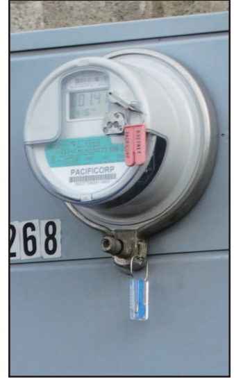
New smart meters will be installed throughout the county by mid-February.
