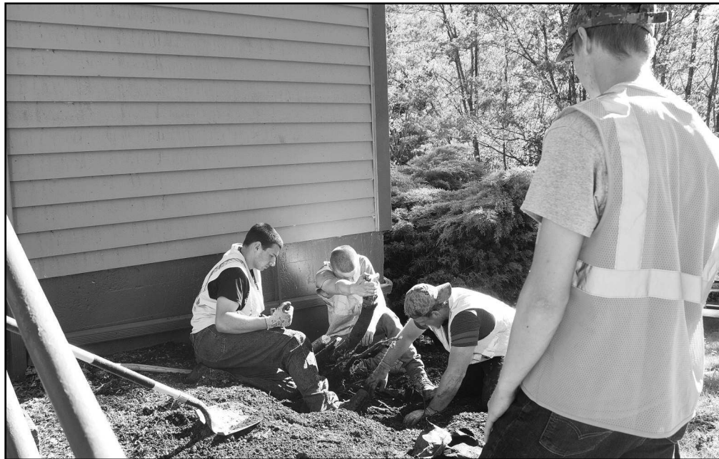
Supervisor Alex Ogden watches as three crew members remove shrub roots.
