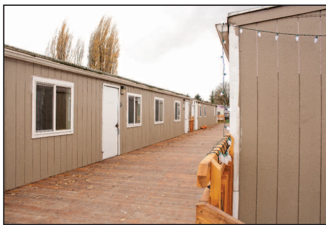
EHCS uses five modular buildings for classes and an office.
