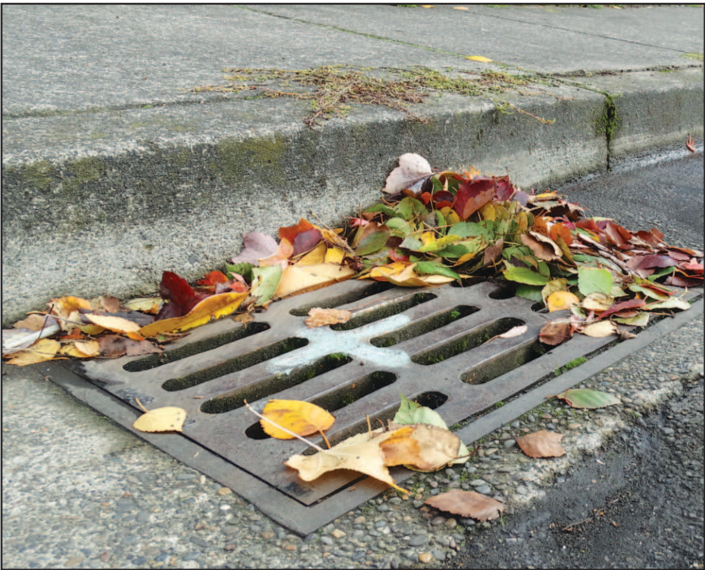
Leaves can clog drains, which can lead to water buildup and localized flooding.
