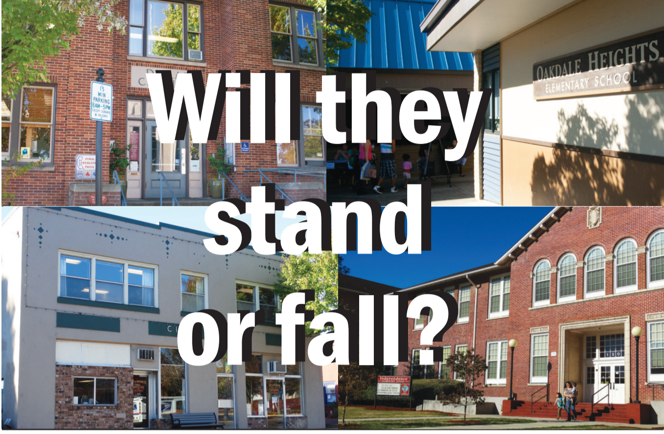
Some buildings — even old ones — will stand during and after a 9.0 earthquake, while others will not. Itemizer-Observer staff
