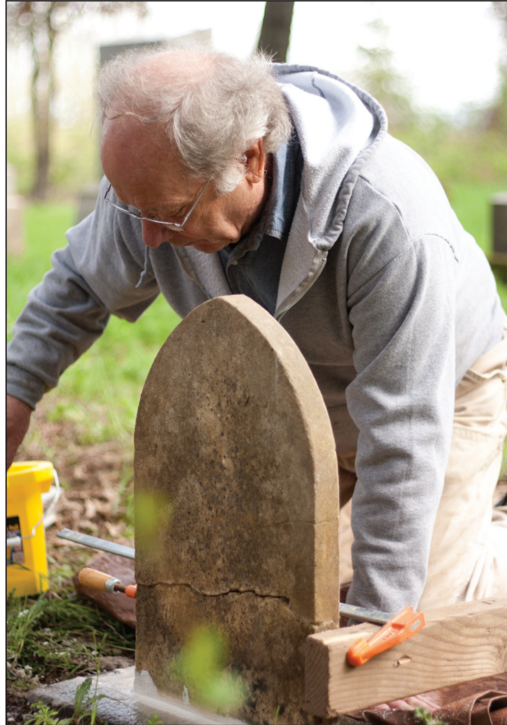
JOLENE GUZMAN/Itemizer-ObsERVER Lloyd Collins repairs a headstone at Chamberlin Pioneer Cemetery during a recent weekend Polk Cemetery Savers work session. The group is in need of more volunteers.
