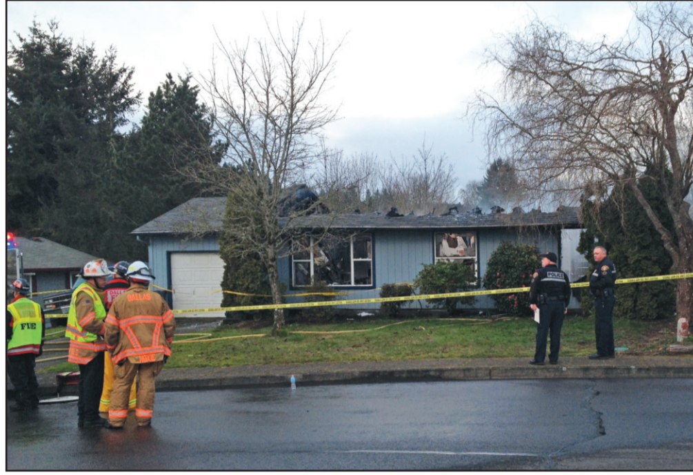
DALLAS POLICE DEPARTMENT/for the Itemizer-Observer Dallas firefighters and police officers monitor what remains of a home on Wyatt Street in Dallas Thursday. Emergency crews found an occupant of the home dead inside.
