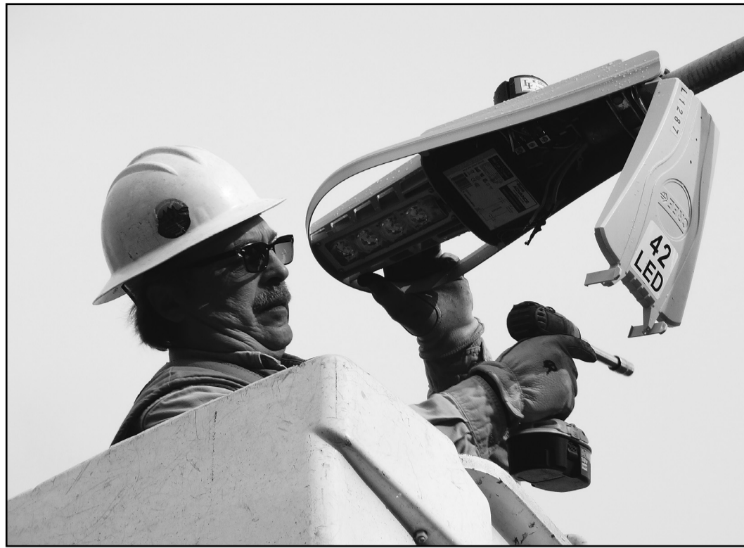
EMILY MENTZER/Itemizer-Observer Russ Downer installs a new LED light on a streetlight in the neighborhood of Candlewood Way. The new lights give off a clearer, whiter light than the old ones, and use less energy.
