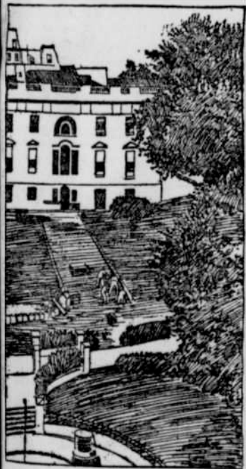
REPLACING FOUNDATION OF EAST WING
