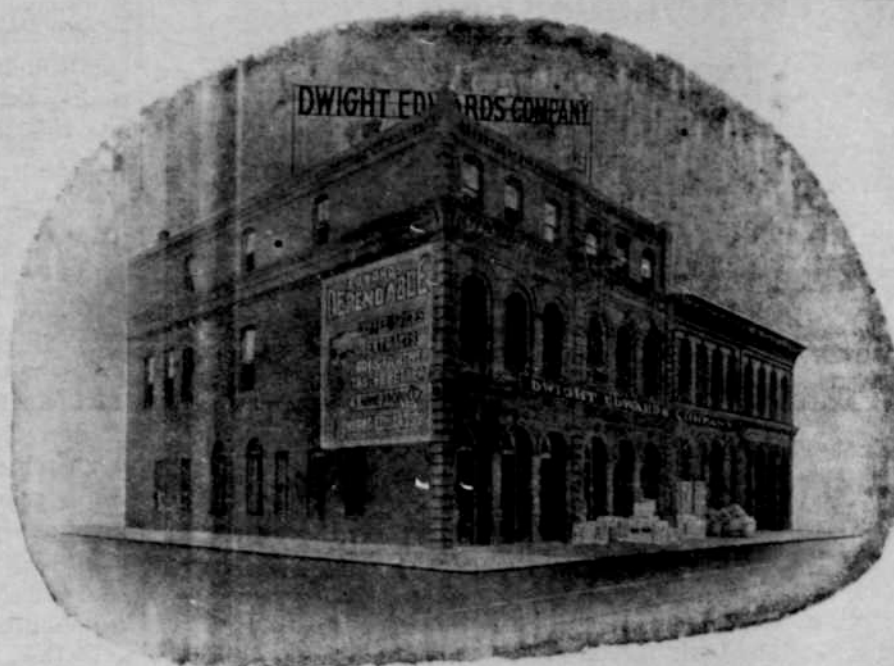
DWIGHT-EDWARDS COFFEE MANUFACTURING PLANT, PORTLAND
