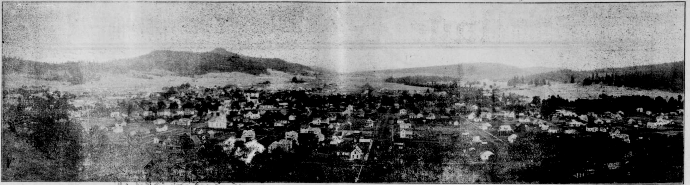
General View of Cottage Grove Looking South From McFarland Hill.
