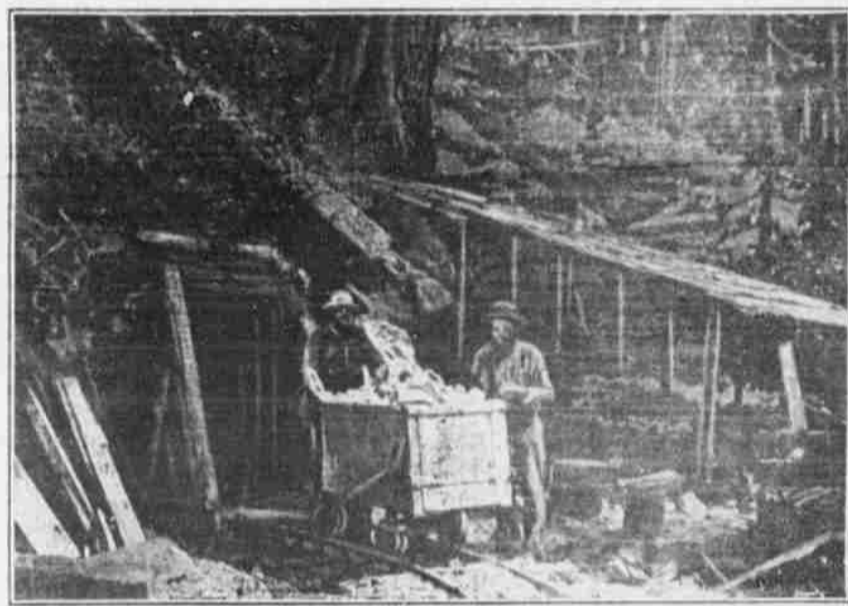
A Bohemia Tunnel.
