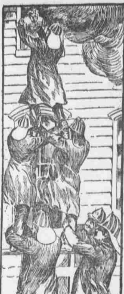
How members of the Chicago fire department reach a high window when the ladder is too short.
