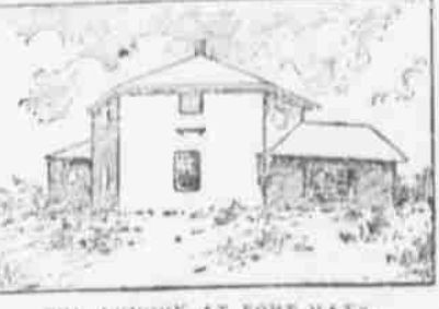
THE ALMS HOUSE AT FORT HAYS.
