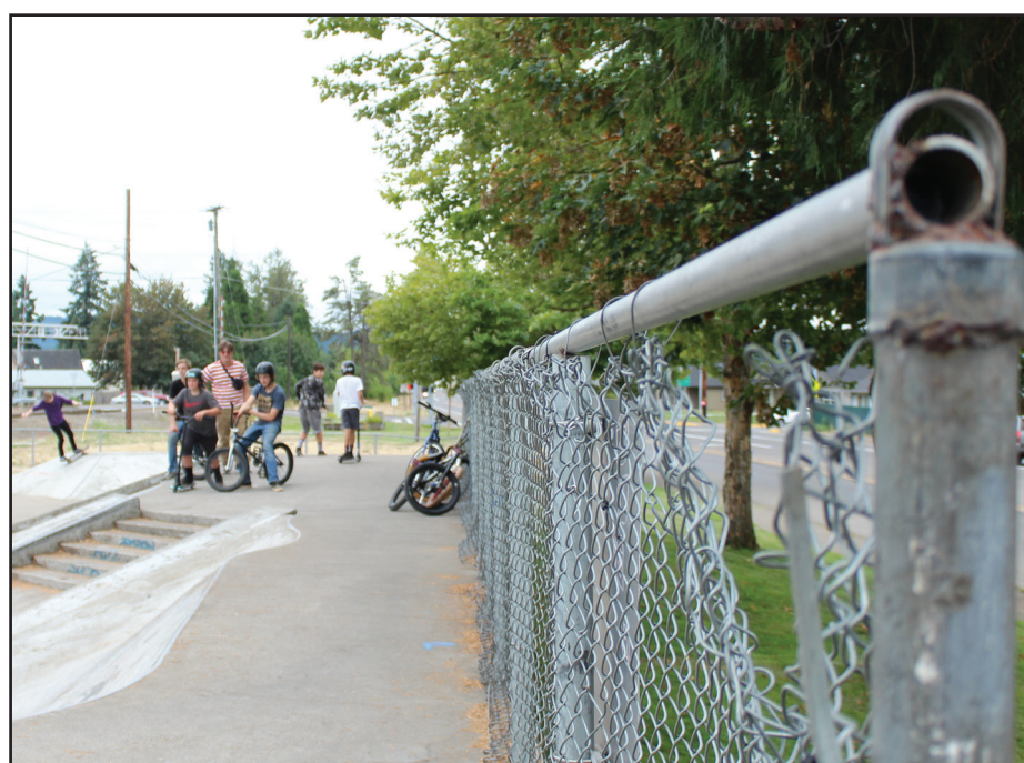
(Top) Graffiti can be seen all over the concrete at CG skatepark, but it doesn't deter most users. (Bottom) The perimeter fence of the park, seen in the foreground, has warped and bent over the years. PHOTO BY NICK SNYDER/CG SENTINEL
