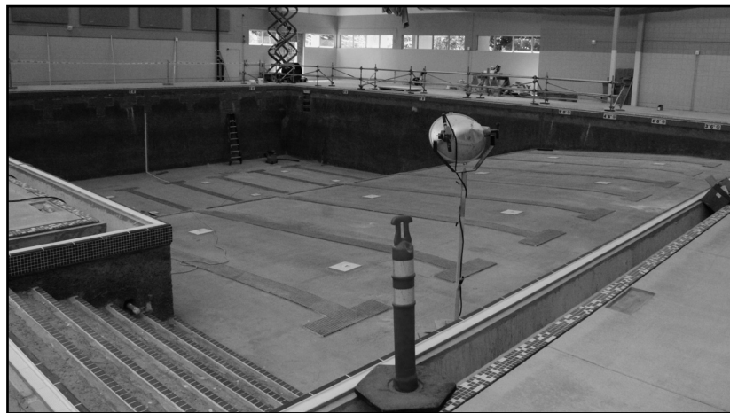
Above: The solar panels soak in the sun outside the Warren H. Daugherty Aquatic Center. Below: The new pool was recently tiled. PHOTOS BY SILVA/CG SENTINEL
