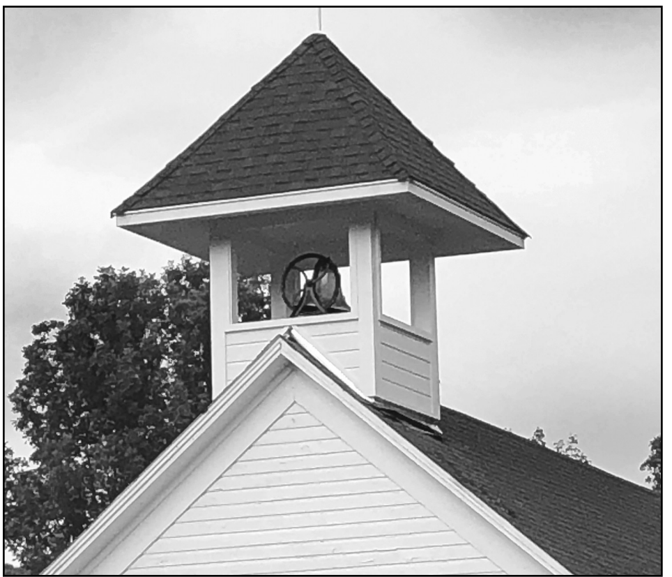
The completed Church at London bell tower, silent for more than a decade, will ring again tomorrow thanks to community efforts.
